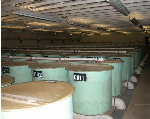
SARL Room 160 Before Renovation
